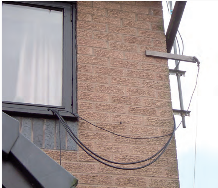
A short run of coaxial cable, from the shack window to the start-point of the antenna wire. The cable’s screen connection is taken to a wire that’s buried under the front lawn.
