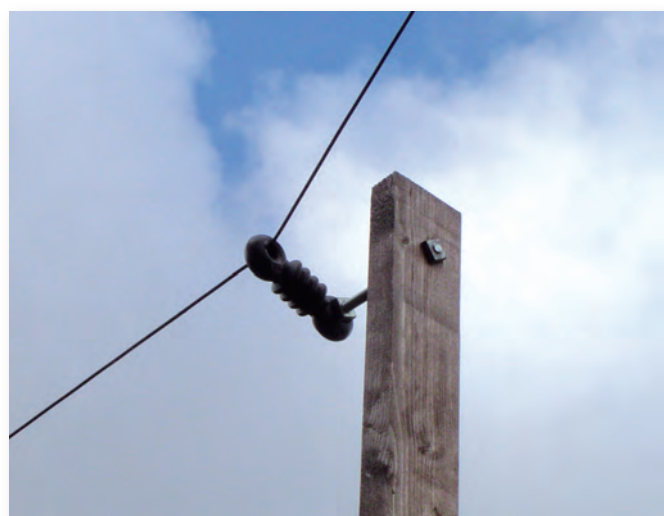
A closer look at the support bolt and the fitted 'dog-bone' insulator.
